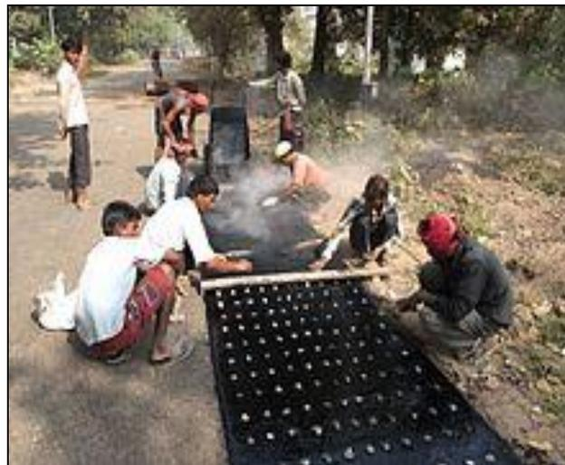
Fig 3: Manual road repair taking place on rural roads
