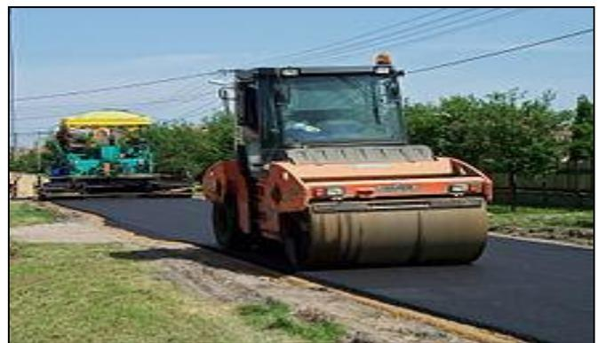
Fig 2: Asphalt layer and Hamm road roller
